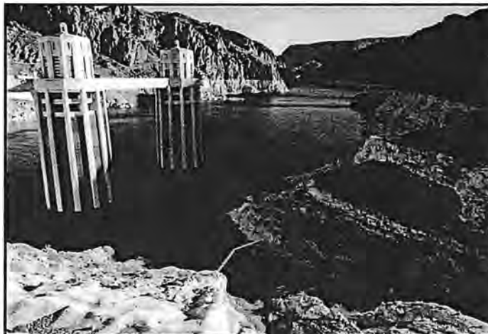
Water intakes on Lake Mead behind Hoover Dam on the Colorado River. Photo by Bureau of Reclamation.
